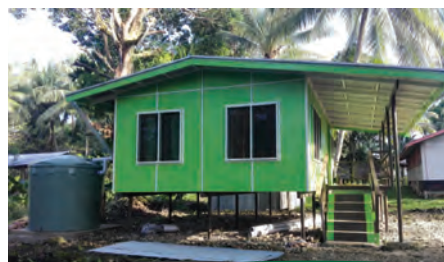
BSP Alotau renovated two Birth Houses and installed water tanks
