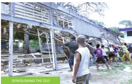
DEMOLISHING THE OLD
