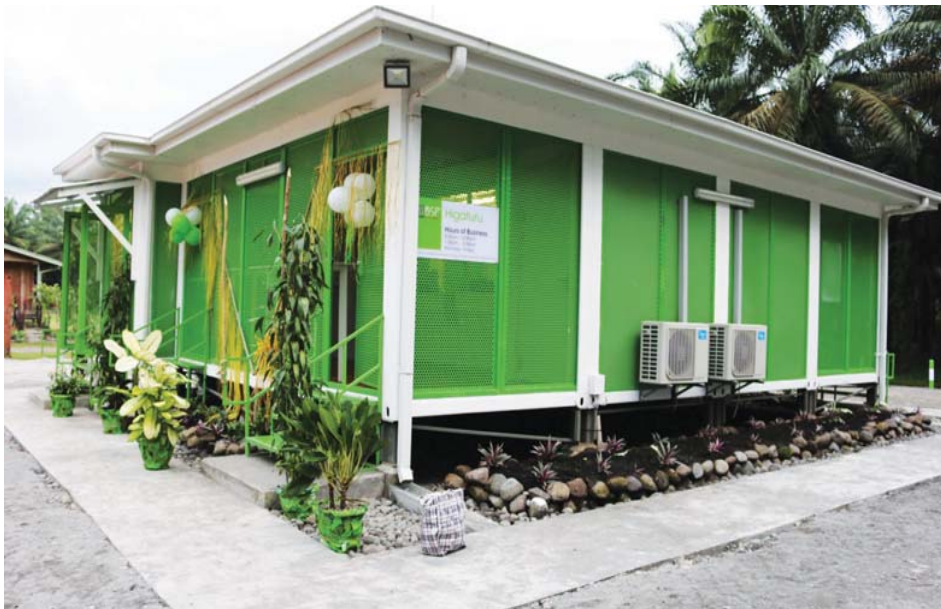
Busy year in construction. Including new Sub Branches. This is the Higaturu Sub Branch in the Northern Province.
